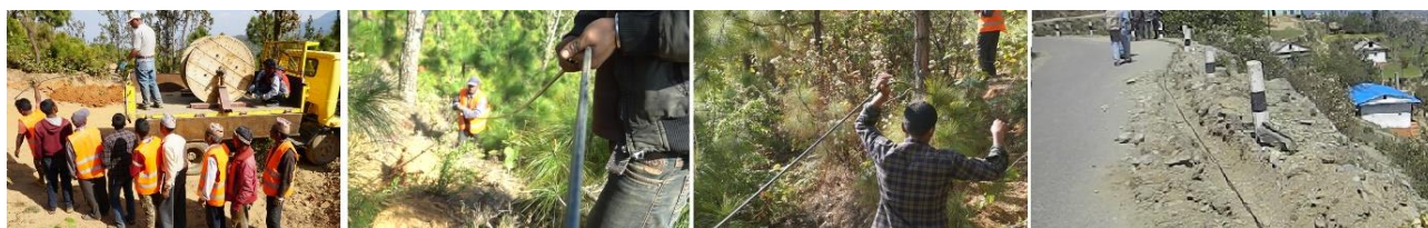
Figure 3. L.110 cable placed on the ground's surface (Jungle) and shallowly buried (roadside)
